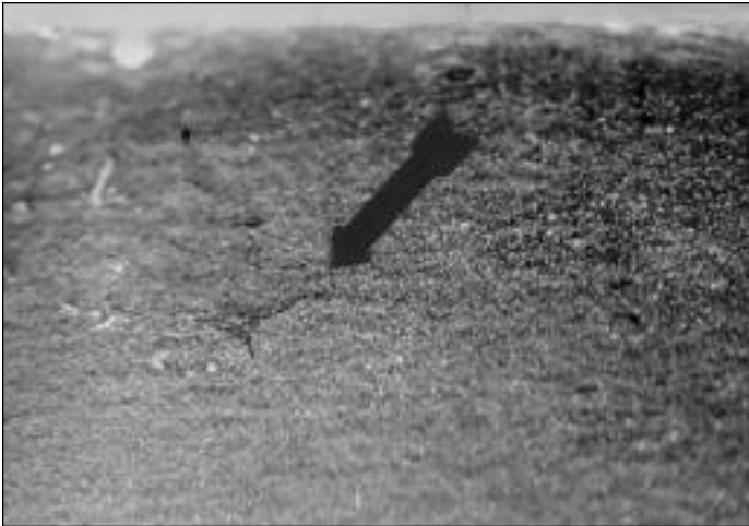
Photo C6. Close-up on bottom side of Tab C-5 at area depicted in Photo C5. Note fracture.
