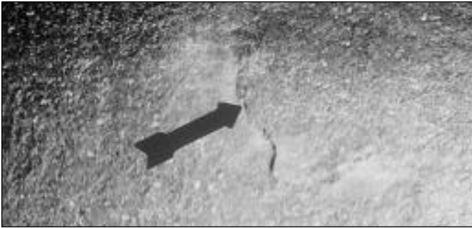
Photo 6. Close-up on bottom side of Tab D-4 of half-panel designation CO-FS-D-7 at impact site. Note curved-line fracture pattern weathered 4 years 4 months.
